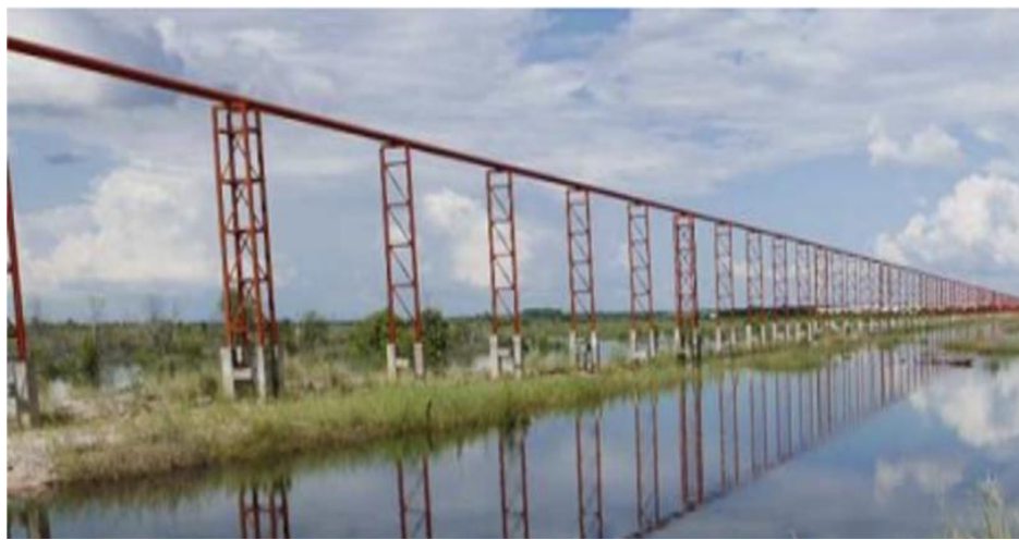
Figure 9. NSSS Direct Piping System at NSP
