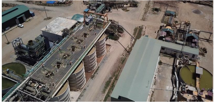
Figure 6. CIL Tanks in Plant 2 (Palu)
