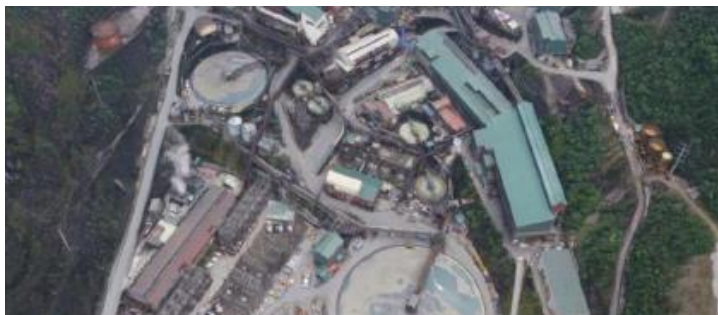
Figure 9. Copper Cleaner Circuit Construction Project
