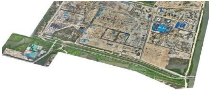
Figure 13. Manyar Smelter Construction Management
