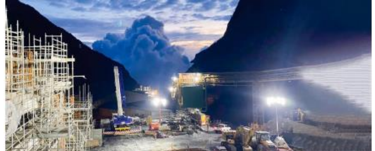
Figure 8. GBC Pre-Crusher Construction Services Project
