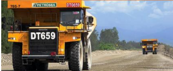
Figure 7. Levee Construction & Stockpile Project
