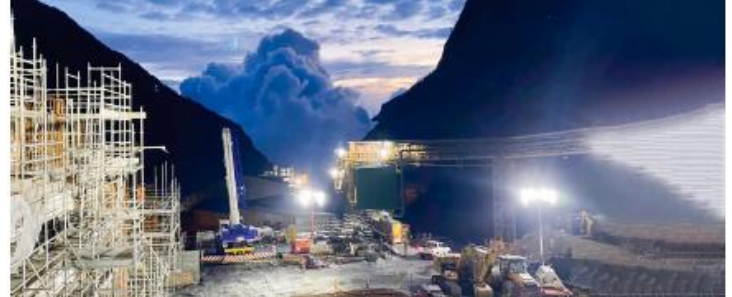
Figure 8. GBC Pre-Crusher Construction Services Project
