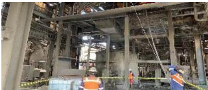
Figure 11. Portsite Corrosion Project
