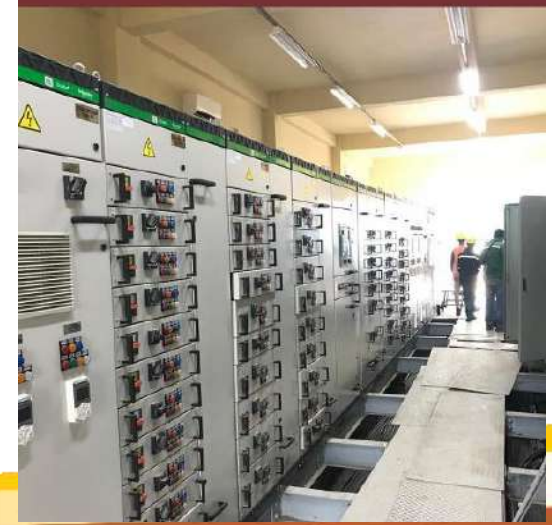
switch gear room for low voltage electricity
