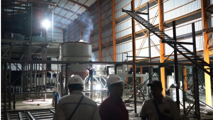
Figure 1. NSSS' 2 nd Palm Oil Mill Progress
