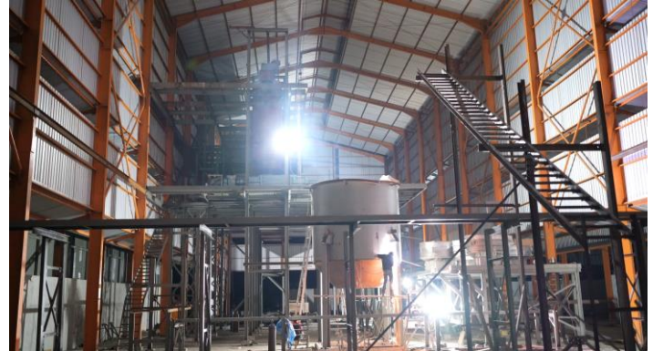
Figure 2. NSSS' 2 nd Palm Oil Mill Progress
