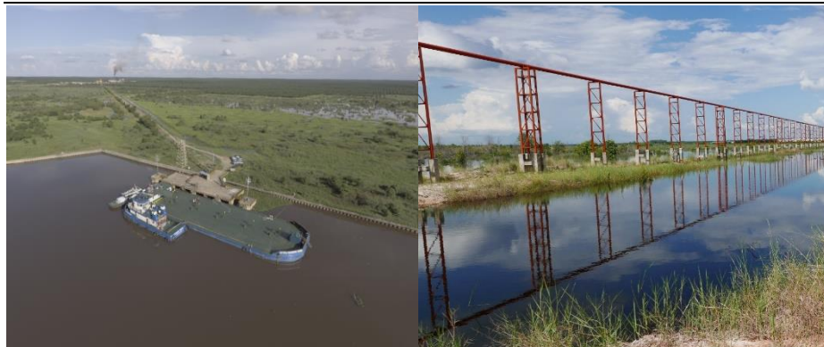
Figure 4. Special Terminal and CPO pipe transport system
